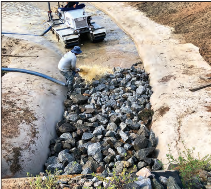
A combination of dredged sediment and excess fill from the project fills the SOX system and then secured by pound the staking system subsurface.
