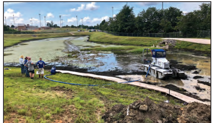
Using an amphibious work boat, pond sediment is dredged into the SOX system to stabilize the shoreline.
